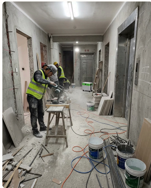
Interior construction power tools operation 室内施工电动工具作业
