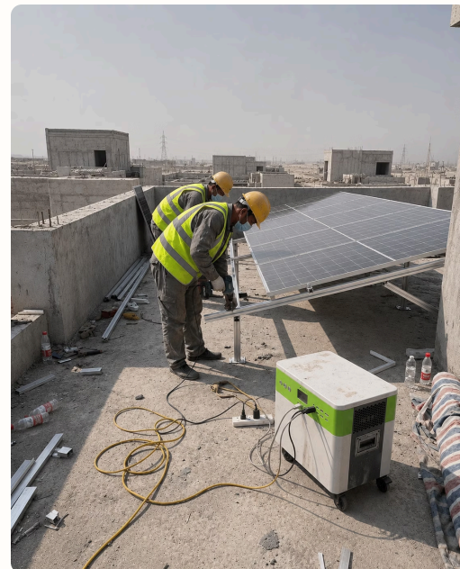
Rooftop equipment installation work 屋顶设备安装作业
